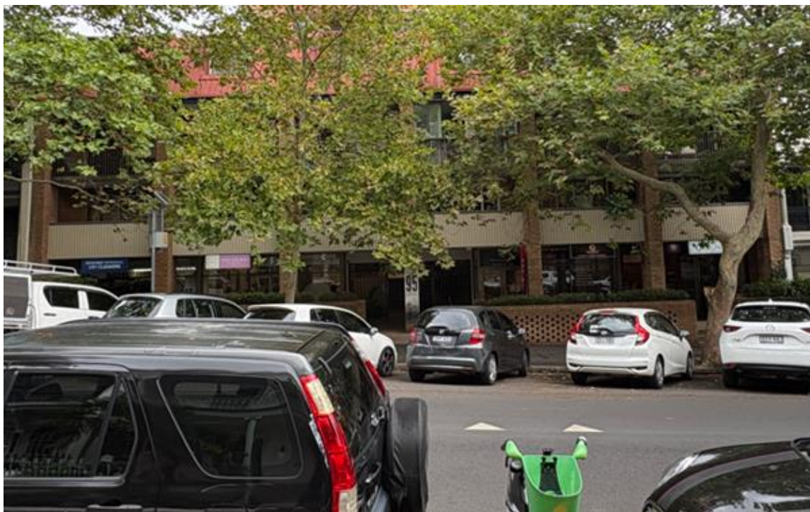
Figure 1: 95 Victoria Street, Potts Point viewed from the east
